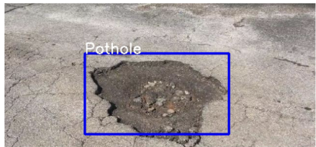
Figure 3: Example of computer-vision techniques applied to pothole detection on road surfaces [7]
