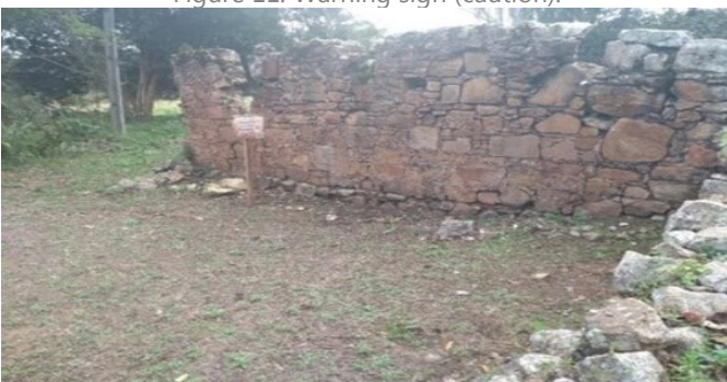
Figure 11: Warning sign (caution).
