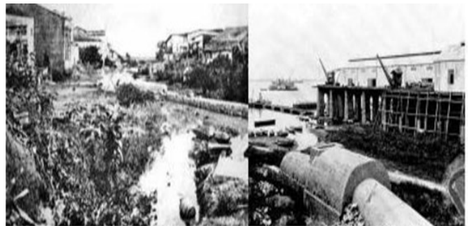
Figure 1 - Drainage of the Espirito Santo creek (left) and galleries built before paving near the Manaus Port area (right) between the years 1892-1900
