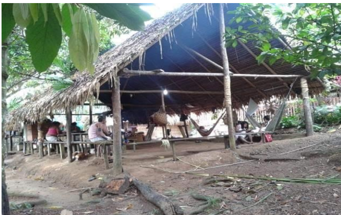
Figure 5: Shed where the community kitchen is located.
