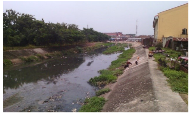
Figure 7 - a) Adequate setback and concretized canal channel behind the University of Lagos. b) Encroached canal setback by a religious organization (the yellow building) just behind the canal.
